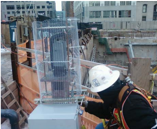
GEI with Automated Theodolite and Weather-proof Data Logger at World Trade Center Site
