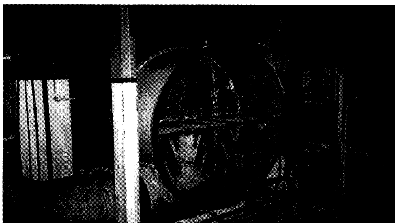
Open end of condenser unit
