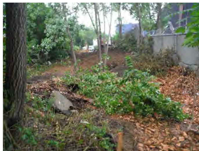
Photograph 6: View of Site during vegetation clearing. Date: August 7, 2017.
