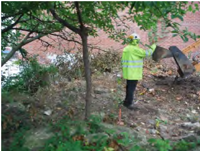
Photograph 3: Site and vegetation clearing activities with a skid steer. Date: August 7, 2017.
