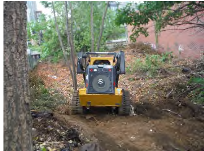
Photograph 4: Site and vegetation clearing activities with a skid steer. Date: August 7, 2017.
