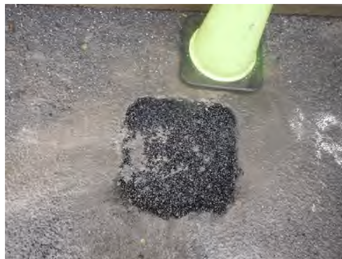
Photograph 22: Asphalt-patch after completion of borehole. Date: August 18, 2017.
