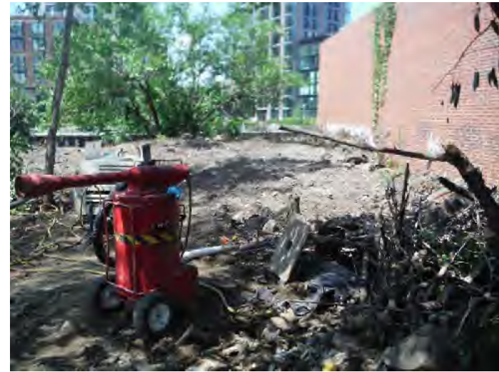
Photograph 12: Air Knife for soft digging activities. Date: August 15, 2017.
