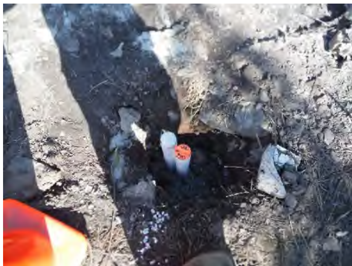
Photograph 29: View of paired groundwater monitoring well prior to installation of protective cover. Date: August 28, 2017.
