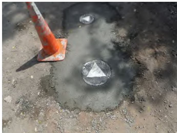
Photograph 31: View of monitoring well MW-3S and MW-3D with flushmount protective covers. Date: August 28, 2017.
