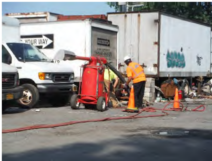
Photograph 13: Performing soft digging activities. Date: August 15, 2017.
