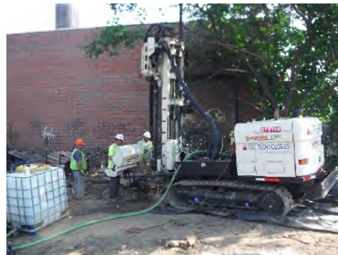
Photograph 20: Roto-sonic drill rig installing well within soil boring SB-6. Date: August 11, 2017.
