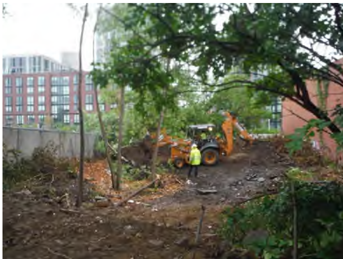
Photograph 5: Site re-grading activities with a back-hoe. Date: August 7, 2017.
