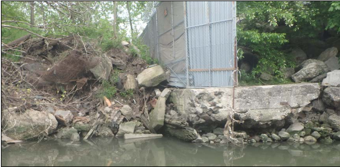
PHOTO 6 – 323 3 RD AVENUE: ERODED RETAINING WALL AT SOUTHWESTERN CORNER OF FORMER FIRST STREET TURNING BASIN
