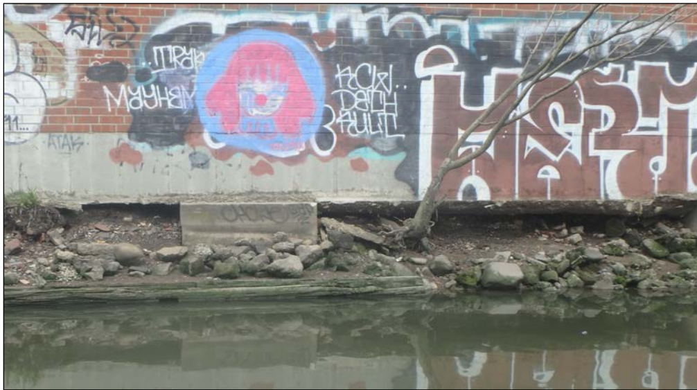
PHOTO 3 – 420 CARROLL STREET BUILDING: UNDERMINING AND MISSING TIMBER PLANKS
