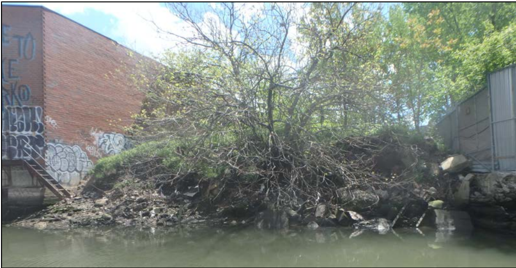
PHOTO 1 – FORMER FIRST STREET TURNING BASIN EARTH EMBANKMENT (LOWER WATER ELEVATION @ 1030 5/9/17)
