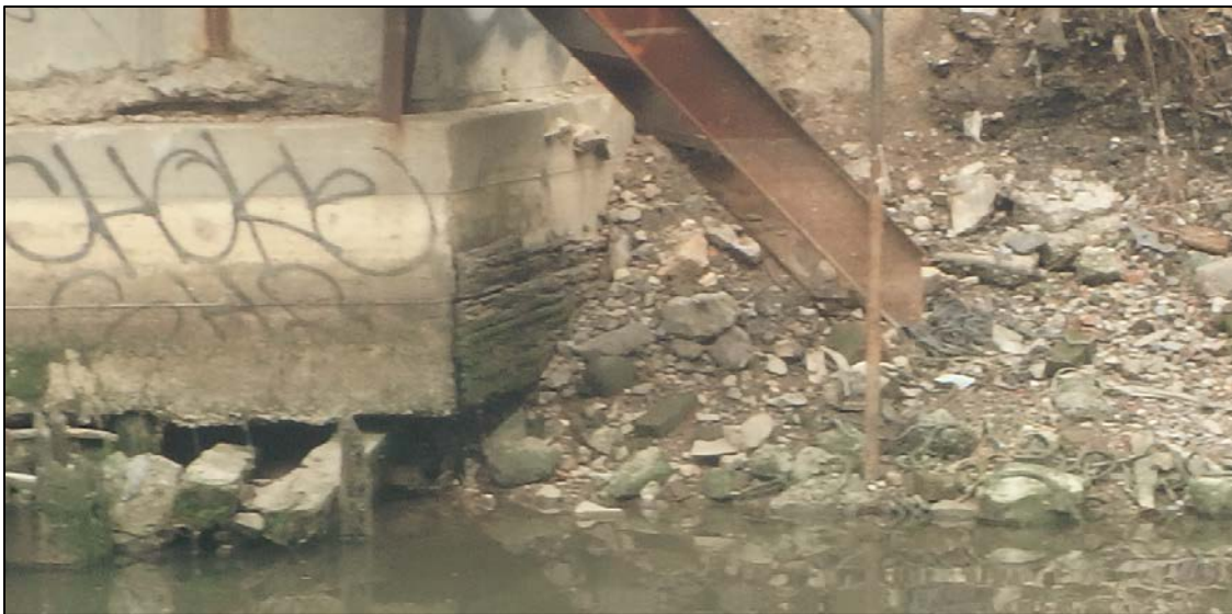
PHOTO 7 – 420 CARROLL STREET: DETERIORATED/MISSING RETAINING WALL AT NORTHWESTERN CORNER OF FORMER FIRST STREET TURNING BASIN
