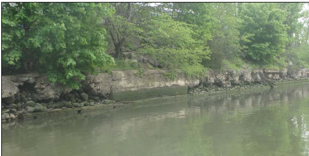
PHOTO 5 – 323 3 RD AVENUE: ERODED CONCRETE SEAWALL AND MISSING TIMBER PLANKS
