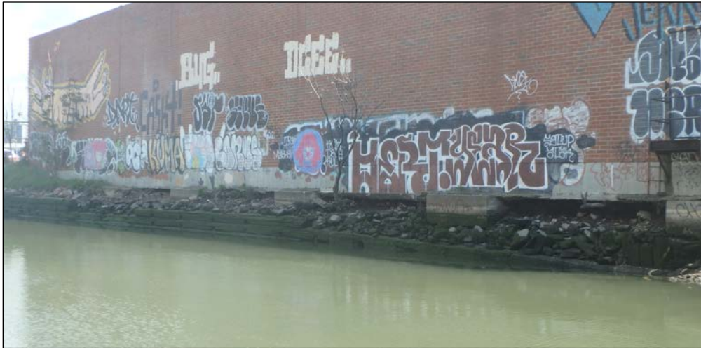
PHOTO 4 – 420 CARROLL STREET BUILDING: UNDERMINING AND MISSING TIMBER PLANKS
