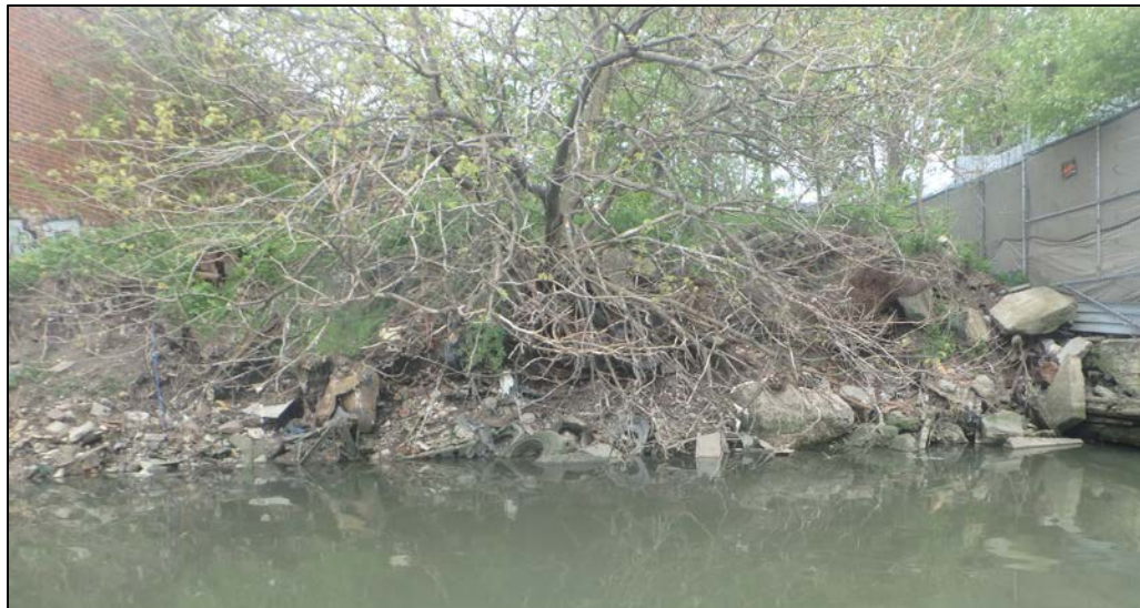
PHOTO 2 – FORMER FIRST STREET TURNING BASIN EARTH EMBANKMENT (HIGHER WATER ELEVATION @ 1630 5/9/17)
