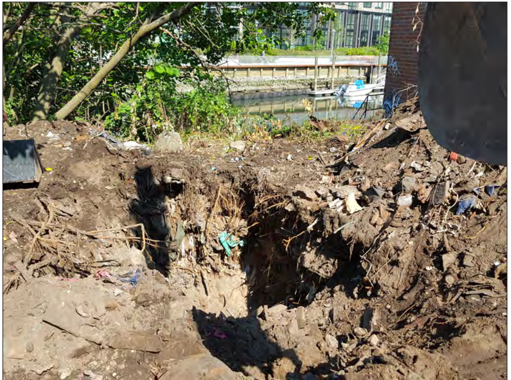
Facing west showing completed excavation of TP1. Note loose sandy fill and extensive modern refuse. The Gowanus Canal is in the background.
