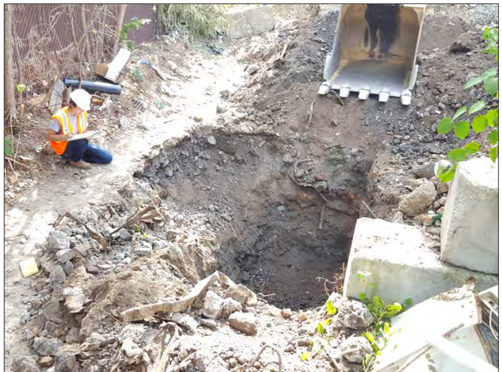
Facing east showing partially excavated TP4. Note loose sandy fills and modern refuse.
