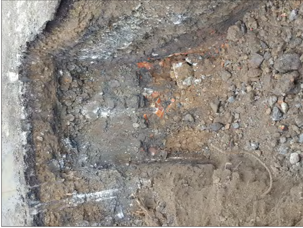
15 Facing south into partially excavated TP3. Note multiple layers of fill and brick demolition debris.
