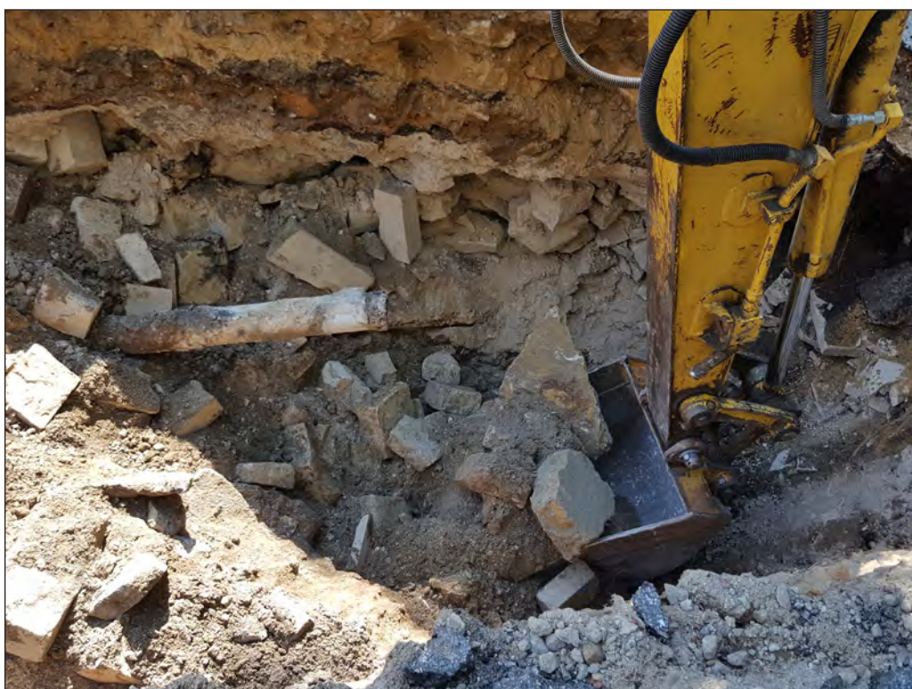
Facing west showing lower portion of western wall of TP6. Note multiple layers of loose fill and demolition debris. Note 6-inch diameter pipe extending into trench from the left. Base of trench is approximately 10 feet below grade in this photograph. 24
