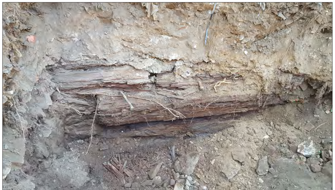
Facing south in TP2 showing portion of wooden bulkhead and fasteners beneath decomposing concrete wall approximately 5 feet below base of fence. Three separate horizontal squared timbers are visible. Base of trench is approximately 9 feet below ground surface.
