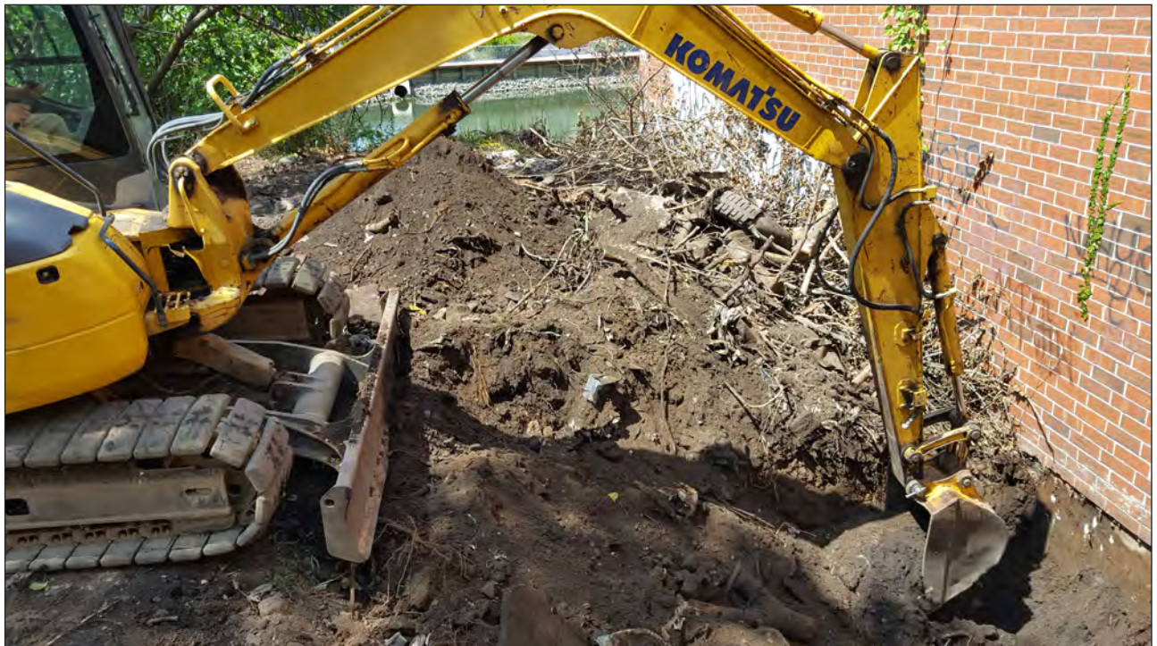
Facing west towards Gowanus Canal showing excavation of TP5 at base of brick building on right. 20
