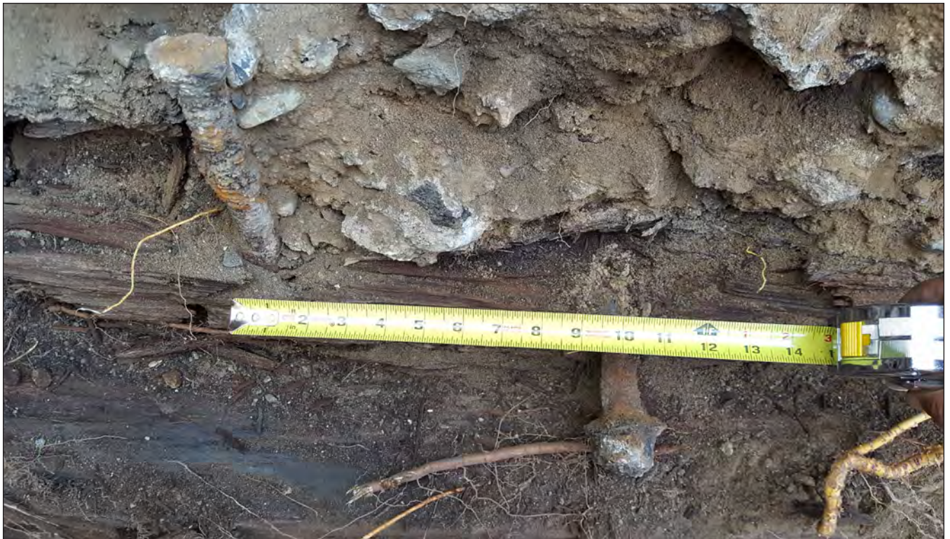
Detail of metal fasteners extending into wooden bulkhead in TP2, immediately below decomposing concrete wall.
