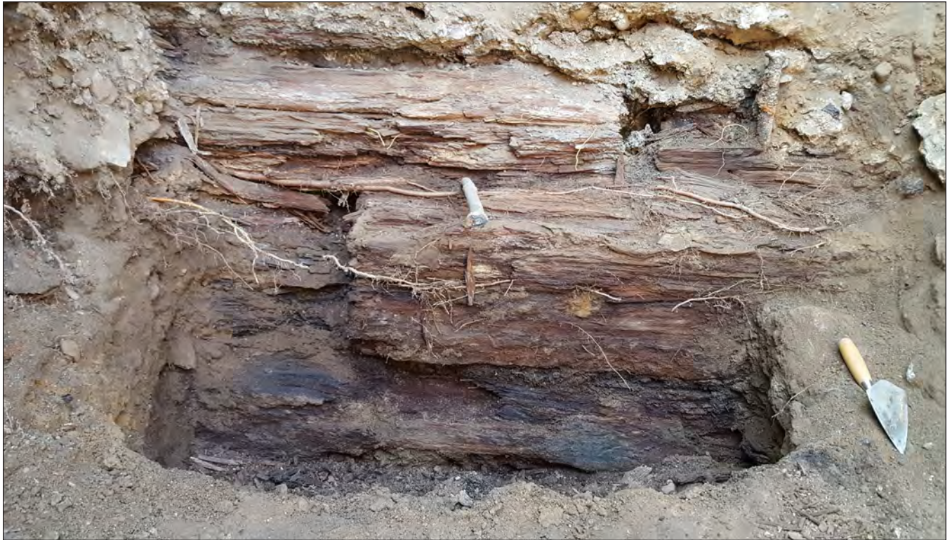
Facing south in TP2 showing portion of wooden bulkhead and fasteners beneath decomposing concrete wall approximately 5 feet below base of fence. Three separate horizontal squared timbers are visible.
