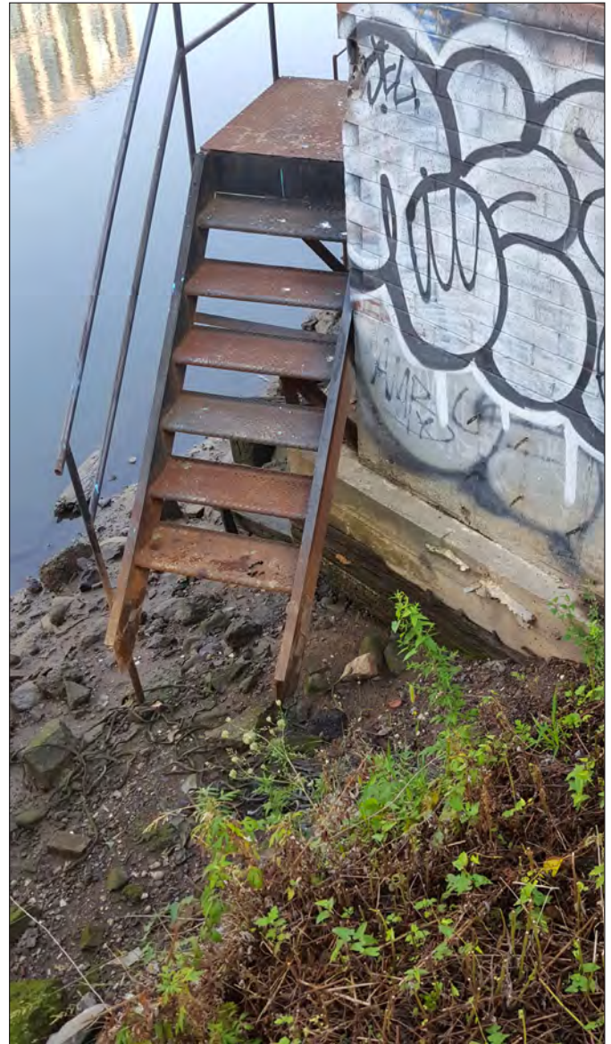
Facing northwest towards foundation of brick building located adjacent to northern edge of basin at its western end. Building is supported by a concrete foundation with a wooden fender.
