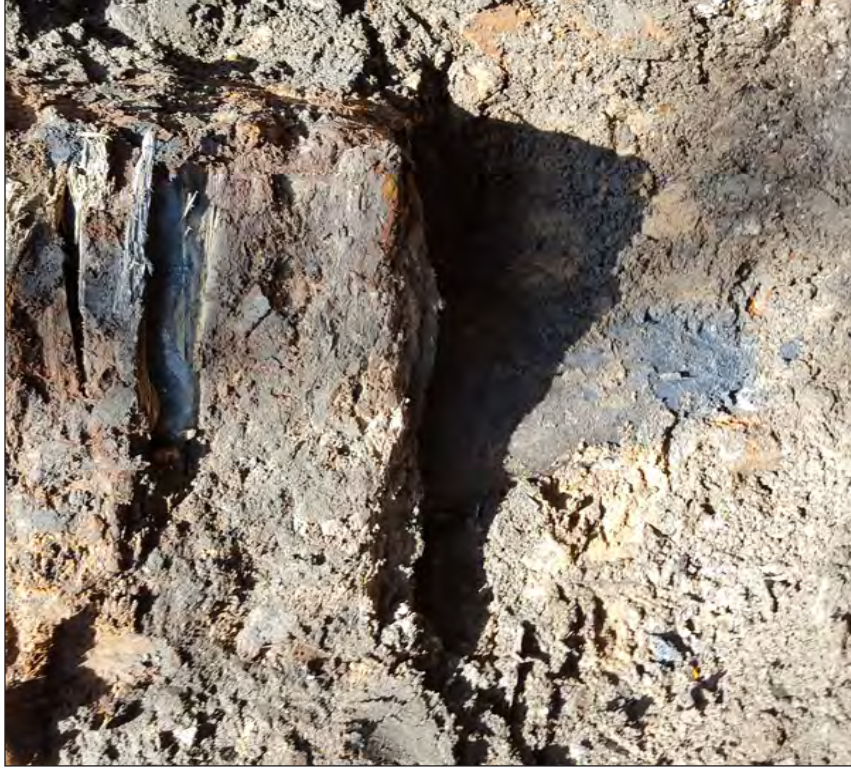
22 Facing northwest at building foundation at northern side of TP5 showing timber pile that is supporting the concrete footer. Soils at bottom of photo are approximately 6.5 feet below base of brick building.
