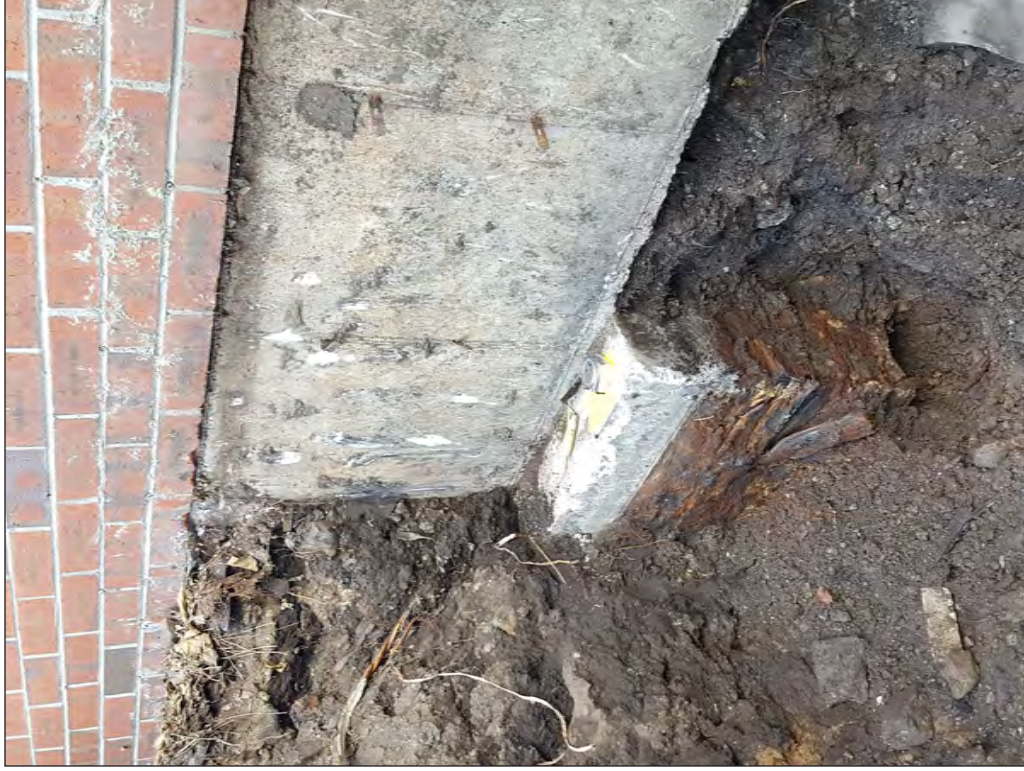
21 Facing northwest at building foundation at northern side of TP5. Brick building is resting on a concrete foundation supported by a concrete footer within a matrix of mixed fill. Remains of the wooden form used to pour the concrete footer are still present.
