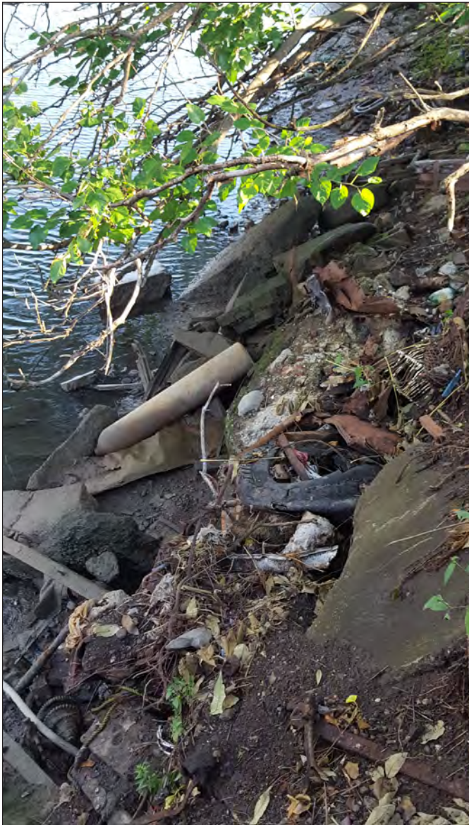
Facing north along the western edge of the filled-in 1st Street Turning Basin showing accumulated debris, loose soils spilling into the canal, and the absence of a retaining wall.
