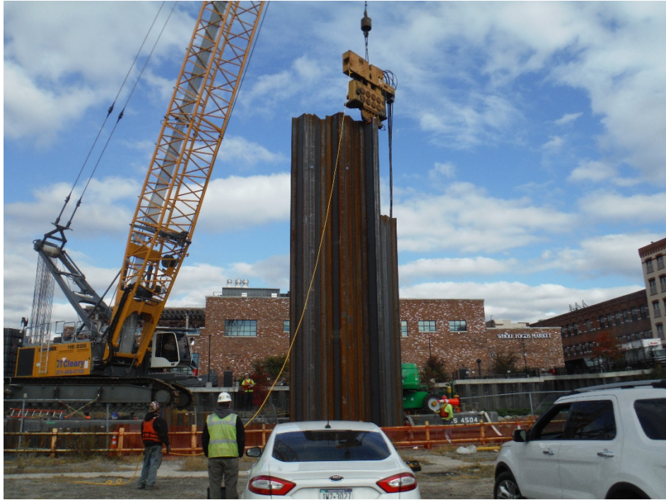
Figure 6. Example of Panel Pile Driving
