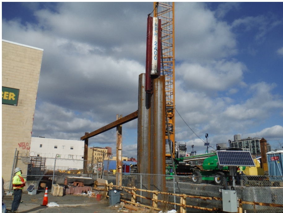
Figure 5. Example of Impact Hammer Pile Driving
