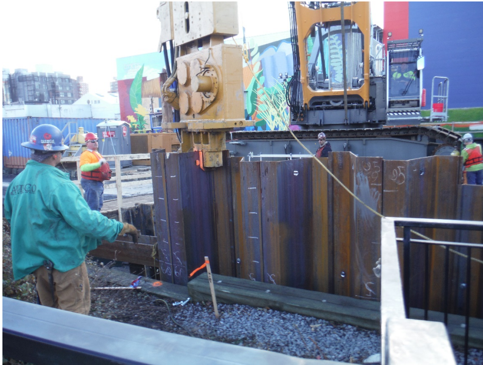
Figure 7. Example of Pitch and Drive Pile Installation
