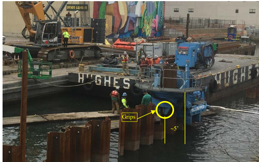
Figure 1. Photo of Giken Set on Sheet Pile
