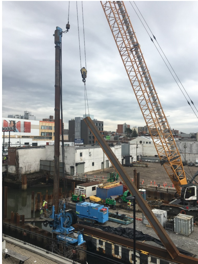
Figure 3. Photo of Crane Lifting Sheet Pile while Holding the Auger
