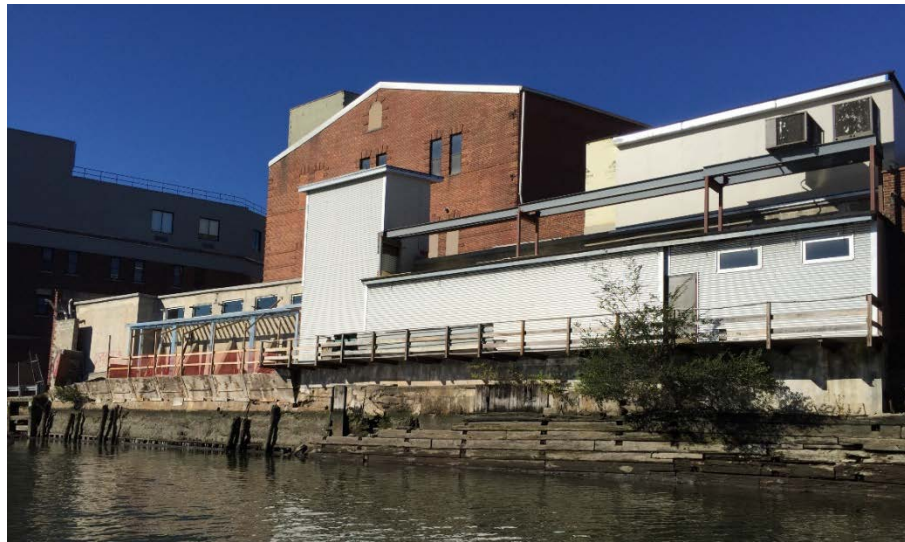
Figure 2. Photo of Property in RTA2 with Structure Immediately on and Cantilevering over Existing Bulkhead
