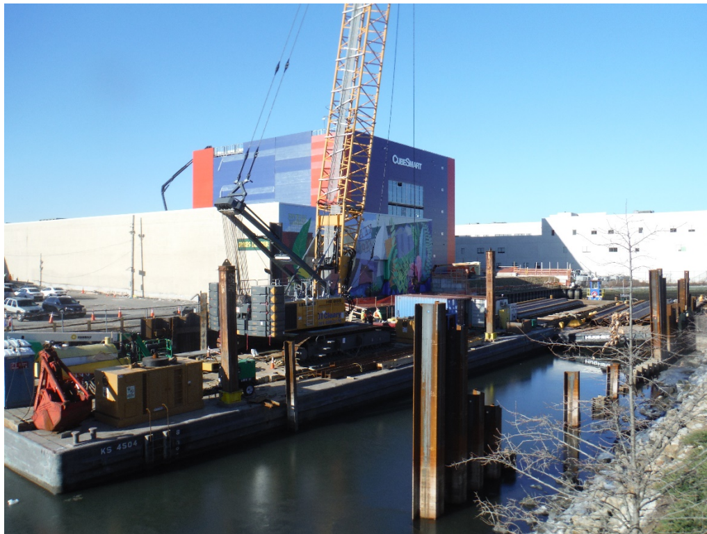
Figure 8. Photo of the Crane and Barges Necessary to Perform the Sheet Pile Installation
