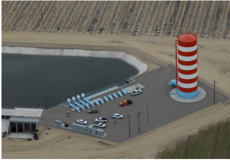
1. 50 Years of Water Resources Planning and Management, Semitropic Water Storage District .
