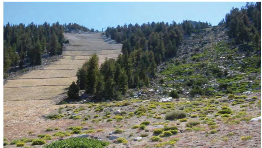
*Side-by-side runs at Mt. Rose Ski Tahoe illustrate the two methods of cutting a run—the one on the left was graded by bulldozer and the other cleared by chainsaw.*
